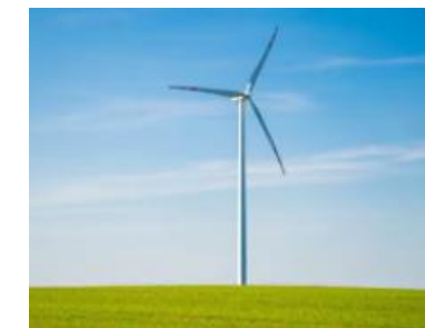
Solar power, wind power, other
